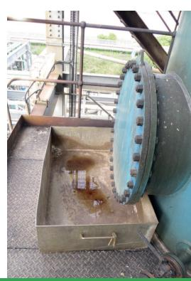
To ensure the optimum level of resources and verification is carried out on each joint, a criticality assessment will be carried out, which will consider the service, pressure and local conditions of each connection.
